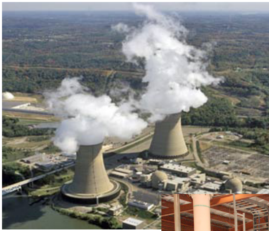
Top: Nuclear power plant cooled with brackish groundwater. Source: U.S. Nuclear Regulatory Commission. Right: Brackish water desalination facility in Harlingen, Texas. The plant was built in 2007 and has a capacity of 2.25 million gallons per day. Source: North Cameron Regional Water Supply Corporation.
