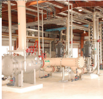
Top: Nuclear power plant cooled with brackish groundwater. Source: U.S. Nuclear Regulatory Commission. Right: Brackish water desalination facility in Harlingen, Texas. The plant was built in 2007 and has a capacity of 2.25 million gallons per day. Source: North Cameron Regional Water Supply Corporation.
