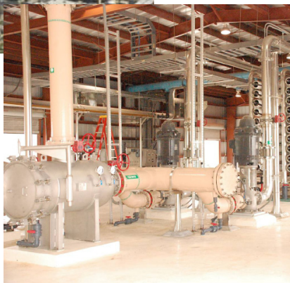
Top: Nuclear power plant cooled with brackish groundwater. Source: U.S. Nuclear Regulatory Commission. Right: Brackish water desalination facility in Harlingen, Texas. The plant was built in 2007 and has a capacity of 2.25 million gallons per day. Source: North Cameron Regional Water Supply Corporation.
